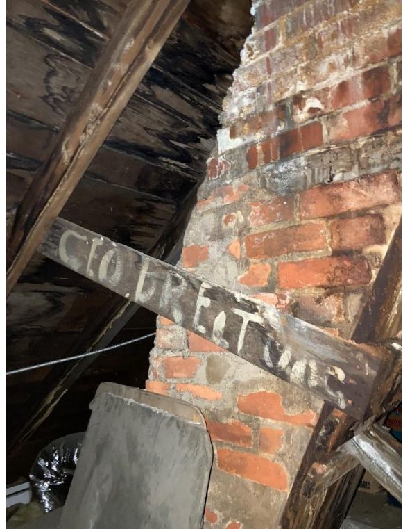
A name in paint across a board in the attic above Teehan's Tavern presents another clue as to whose hands built this historic structure in the middle of the 19 th Century.
